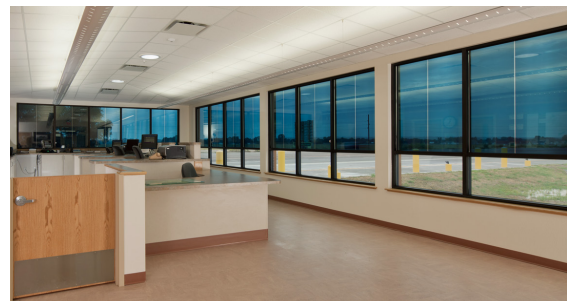
Above: The employee cafeteria in the Siemens wind turbine nacelle manufacturing plant in Hutchinson, Kansas. Below: Port of Entry, Torrington, Wyoming. Both sets of photos show the glass in its fully tinted state (<2% VLT) and in its clear state (62% VLT).
