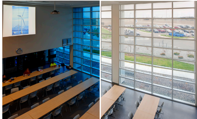
Above: The employee cafeteria in the Siemens wind turbine nacelle manufacturing plant in Hutchinson, Kansas. Below: Port of Entry, Torrington, Wyoming. Both sets of photos show the glass in its fully tinted state (<2% VLT) and in its clear state (62% VLT).
