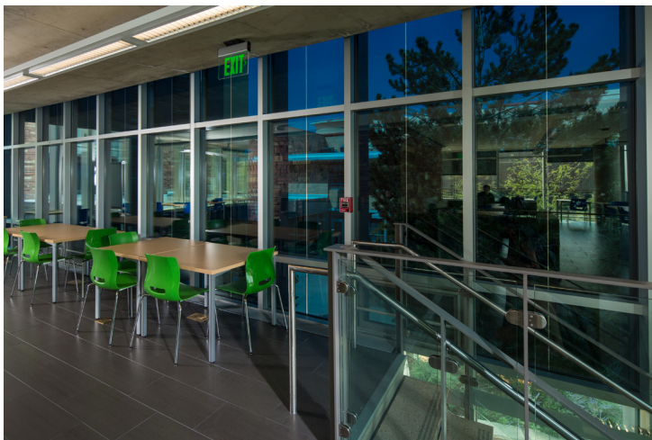
Figure 1. EC glass installed in the Morgan Library expansion at Colorado State University shown in its fully clear and fully tinted states.
