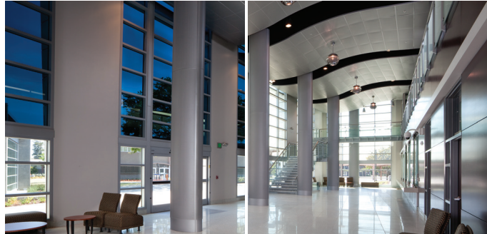
The Student Services Center at Chabot Community College shown with EC glass in its tinted state (left) and clear state.
